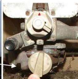
**Lower the thermostat to a temperature you are comfortable with.**
