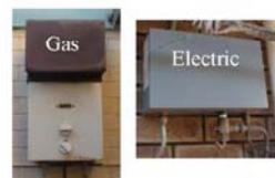
Note that **electric instantaneous systems cannot be turned down**. They are big users of energy when in use, so carefully manage your hot water use.
