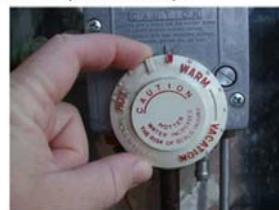
Your water in the storage tank still needs to be hot (at 60 degrees Celsius\*). To test this hold a thermometer under the hot water tap nearest your hot water unit half-a-day after making the adjustment. Check whether you need to adjust it up or can lower it further.
