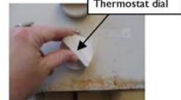
Systems with dials may have two controls– one for ignition and/or flow and one for temperature – you want to lower the one for temperature – typically the bottom control.
