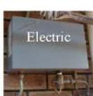
Note that **electric instantaneous systems cannot be turned down**. They are big users of energy when in use, so carefully manage your hot water use.
