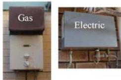
Note that **electric instantaneous systems cannot be turned down**. They are big users of energy when in use, so carefully manage your hot water use.
