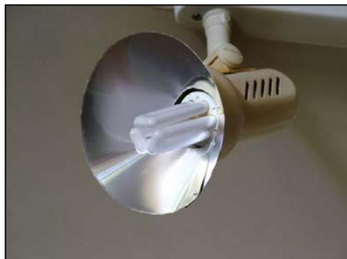
**Figure 5** CFL Lamp with homemade reflector
