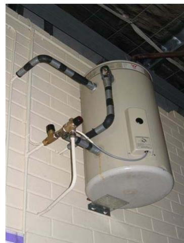
**Figure 7 Pipe insulation on electric HWS**
